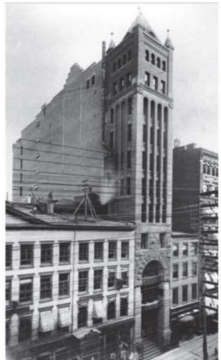
Above, the Tower Building. Gilbert devised the steel-frame construction because of the limitations of a narrow lot.
